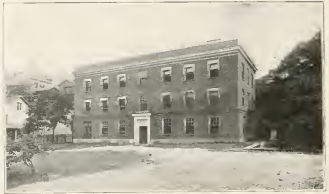
Thirty student nurses are housed in this new residence
